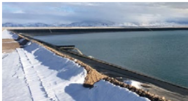
Brine is pumped from the pond underground to tap product.
